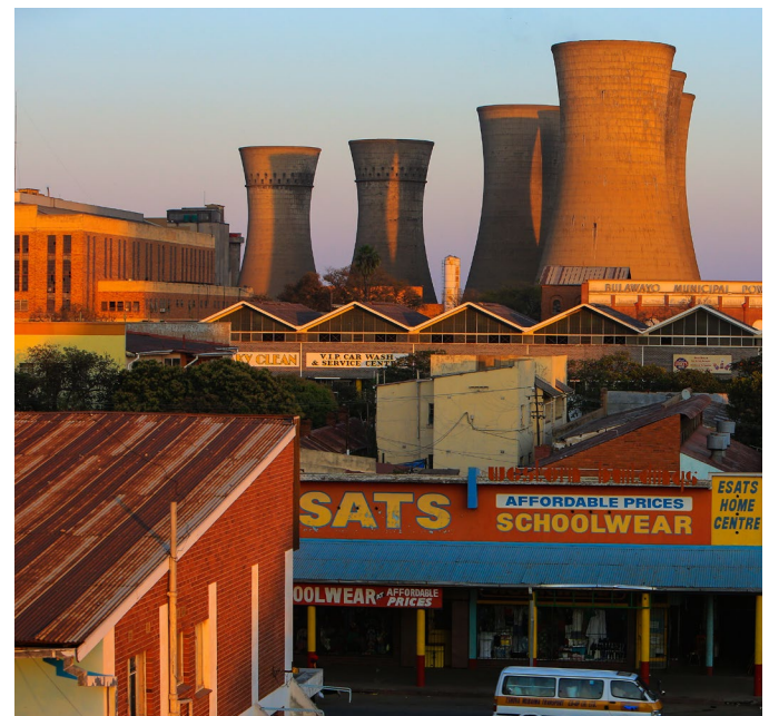
Bulawayo Power Station is a coal-fired thermal plant in Bulawayo, Zimbabwe
